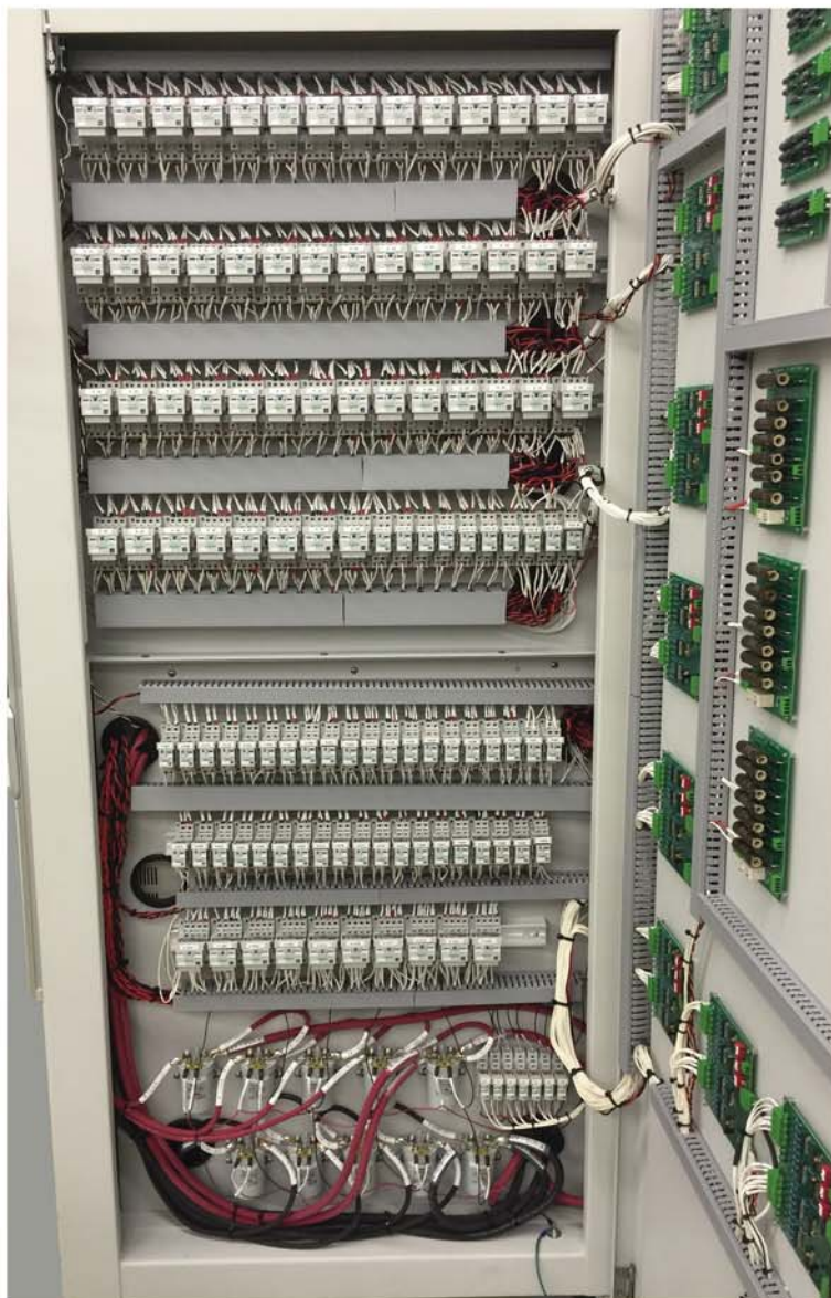
Right-Side Cabinet Extension Open showing over 100 DIN Rail Relays, Relay Drive PCBs, Resistors, High Power Relays, etc.
